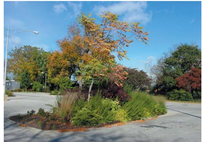
Fig. 1.4 Example of a bioswale in a surface parking lot in Chicago, IL. This treatment uses space that could be otherwise directed towards other uses.
