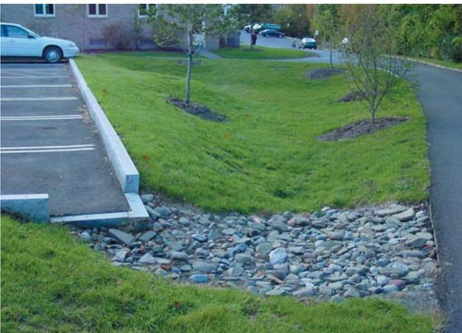
Fig. 1.3 Example of a retention/detention pond adjacent to a surface lot at Cornell University, Ithaca, NY. This treatment uses space that could be otherwise directed towards other uses.
