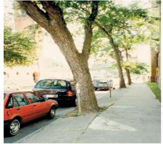
Fig. 1.20 Sidewalk heaving caused by superficial tree root growth, Ithaca, NY
