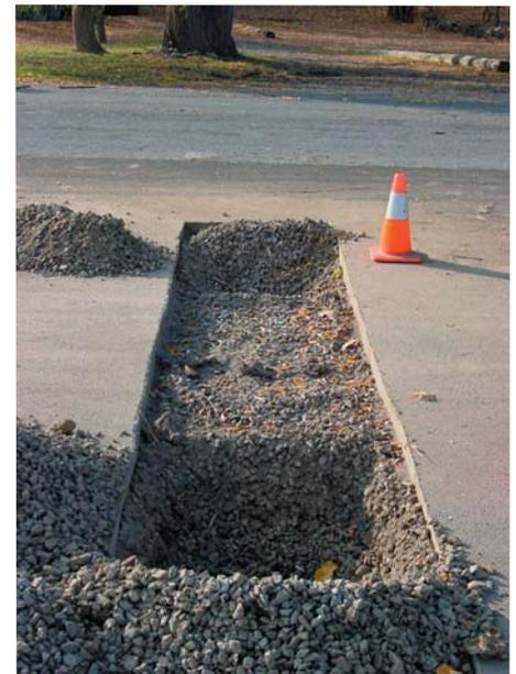
Fig. 1.24 In this parking lot, there is only a 3 foot opening for tree planting. Here CU-Structural Soil® was installed underneath the asphalt to extend the rooting volume for the trees. Once the pavement was cut, bare root Accolade Elms were planted in November 2005.
