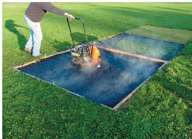
Fig.1.14 Compaction of porous asphalt on CU-Structural Soil® in a test plot on the Cornell University campus.
