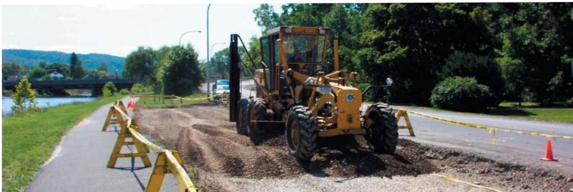
Fig.1.12 Grading of CU-Structural Soil® used as the reservoir base course for porous asphalt lot in Ithaca, NY. For this lot, 2' of CU-Structural Soil® was used to hold a 100 year storm event of 6" in 24 hours.
