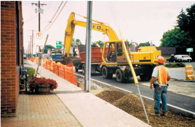
Fig.1.9 Installing CU-Structural Soil™ in Ithaca, NY in 1997
