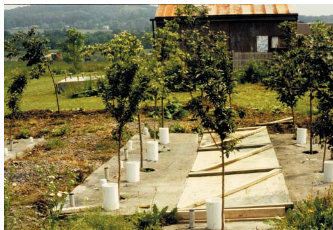
Fig 1.26 In this three-year field study a normal soil profile under sidewalk pavement as well as one with CU-Structural Soil™ were compared. Species used were hedge maple, little leaf linden, and crabapple.
